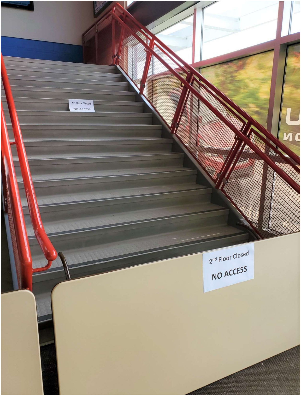
Mezzanine and staircase closed, no second floor access.
